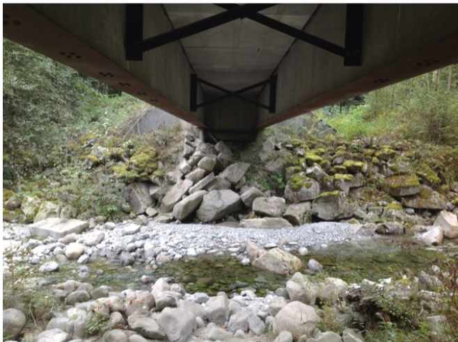
Right Bank Abutment when facing downstream
