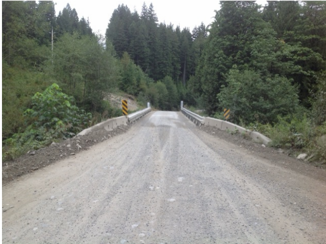
Approach from Right Bank when facing downstream
