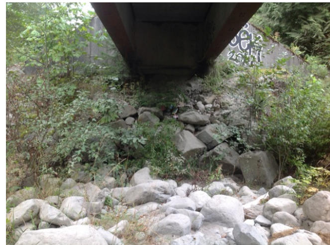
Left Bank Abutment when facing downstream
